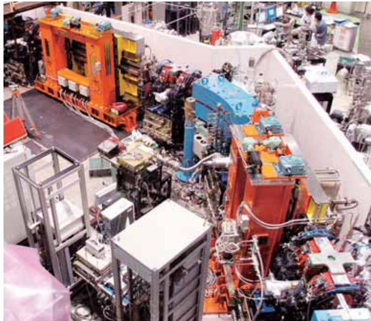
Figure 3 New APPLE-II undulator for BL7U (upper) and In-vacuum undulator for BL6U (lower)
